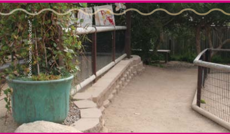
The slope under the fence surrounding the picnic area was removed and replaced with a retaining wall. The retaining wall can be used as a bench for more enjoyable train viewing. Even more updates...
